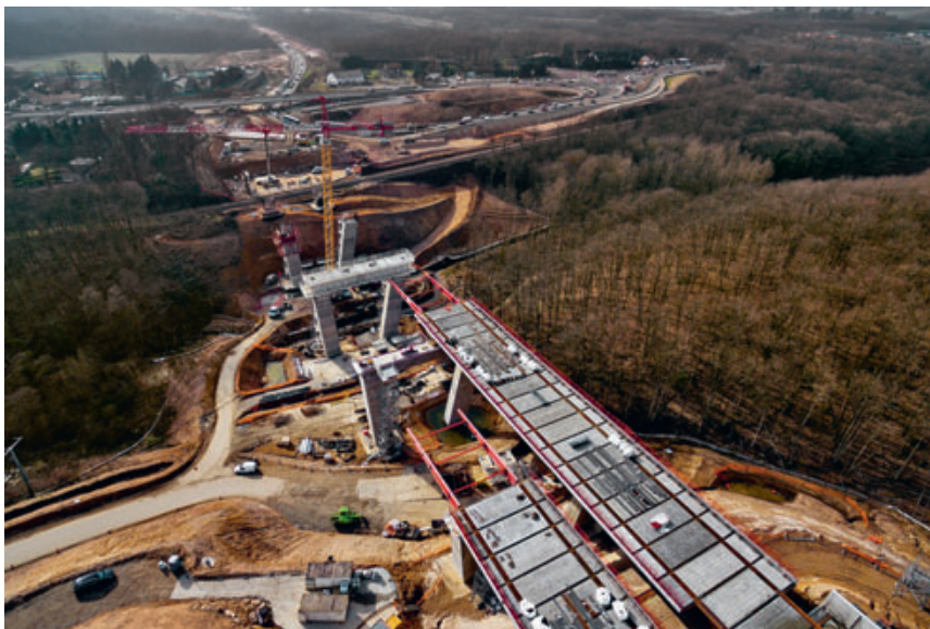
Building the A89-A6 motorway link road
