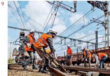
9 Replacing track equipment in Brétigny-sur-Orge.
