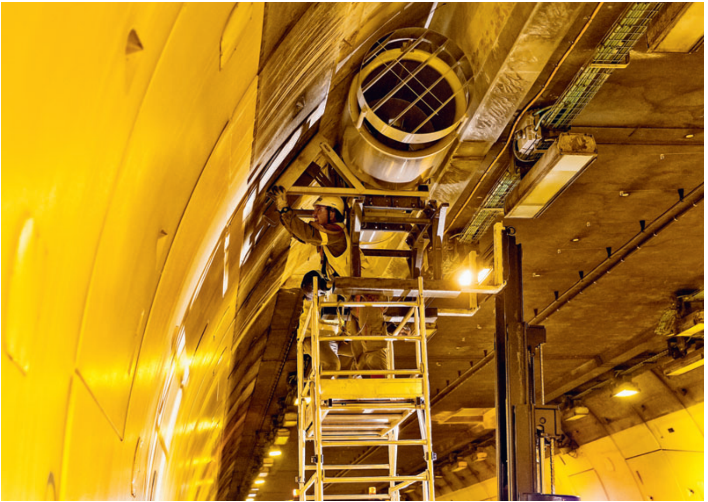
Renovation of the ventilation system in the Caluire tunnel
