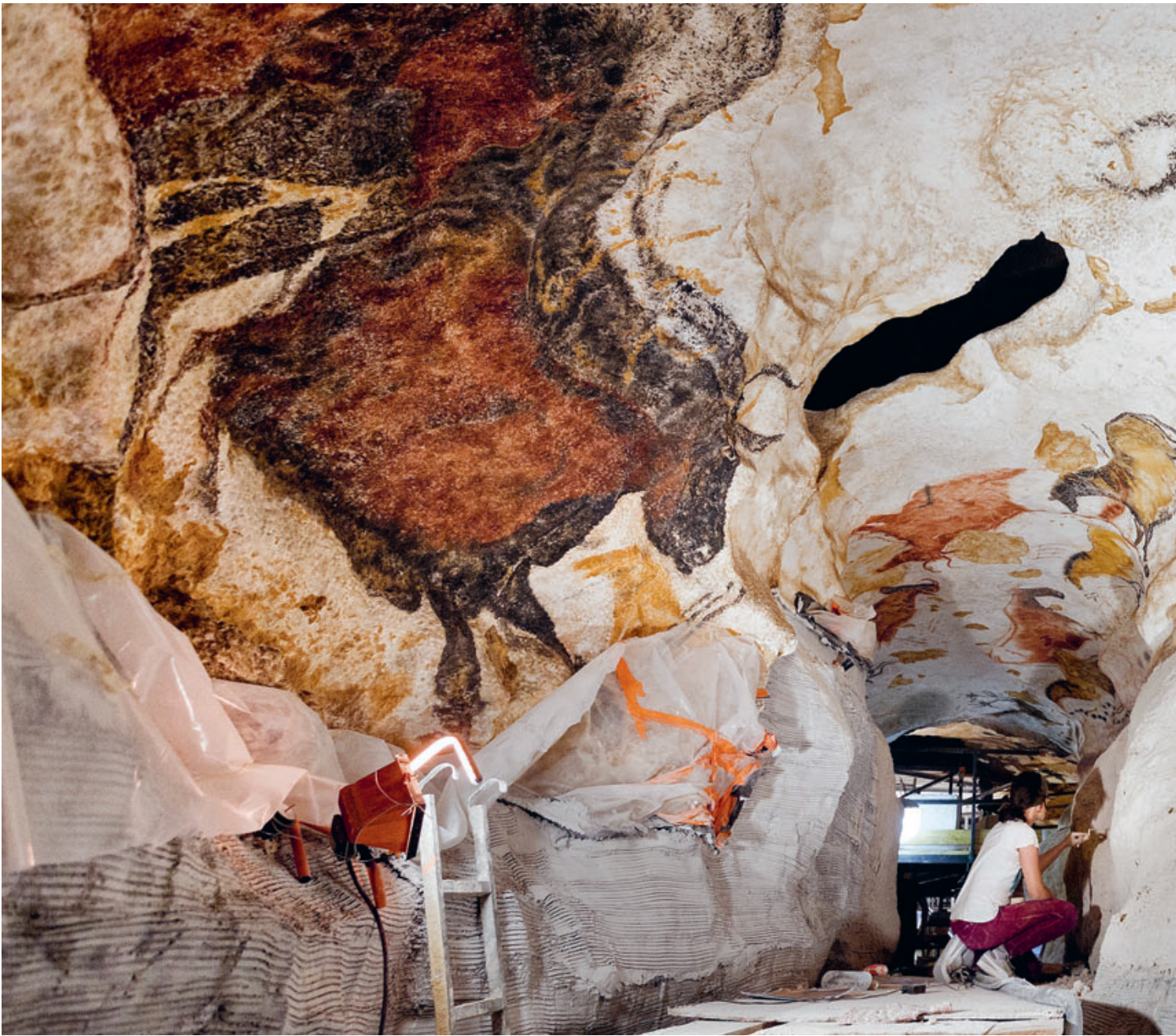
Installing air handling and air conditioning equipment at Lascaux IV, a full-scale reproduction of Lascaux cave in Montignac
